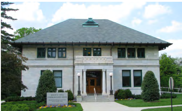
Before: Asphalt shingles on the Visitor Education Center.
