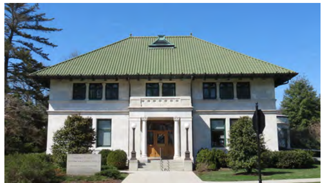
After: The newly-restored Visitor Education Center roof.
