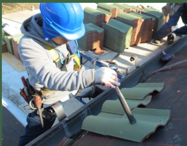
Construction workers from Wagner Roofing place the first new tiles on the roof.
